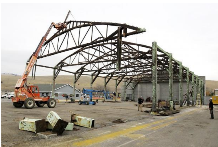
פירוק מבנה. המקור: Keila Szpaller. Missoulain. Company dismantles building at city of Missoula maintenance site for reuse. Nov. 2012. https://missoulain.com/news/local/company-dismantles-building-at-city-of-missoula-maintenance-site-for/article_e1bb32d8-2d41-11e2-8674-0019bb2963f4.html
